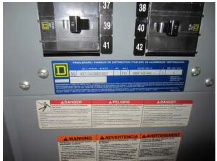
Electrical Distribution Subpanel
