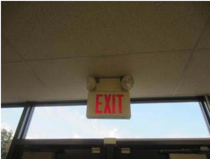
Exit Sign with Emergency Egress Lighting
