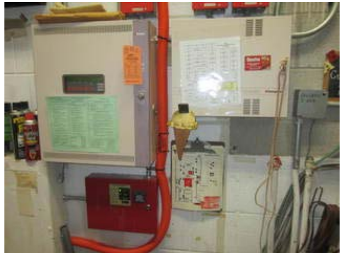
Fire Alarm System Control Panel
