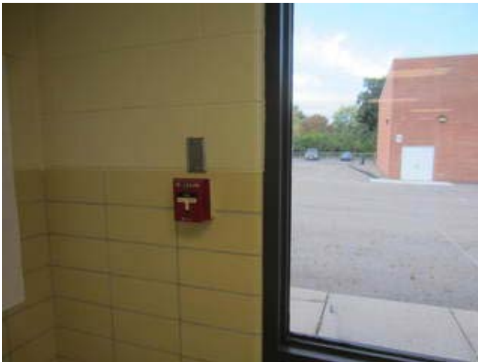
Fire Alarm System Manual Pull Station
