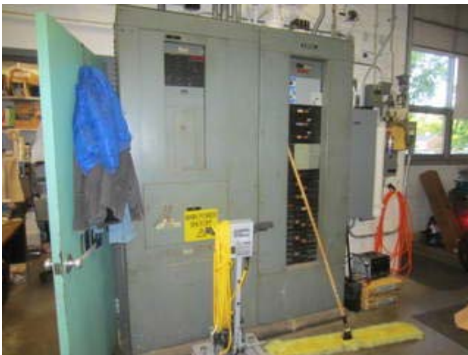
Main Electrical Distribution Panel
