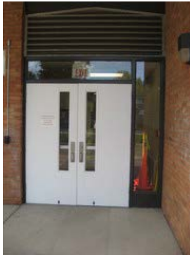
Hollow Metal Door with Transom and Sidelight
