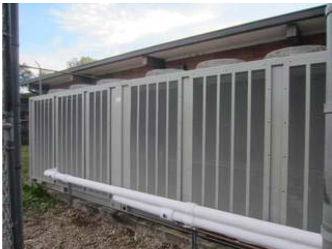
Air Cooled Condensing Unit
