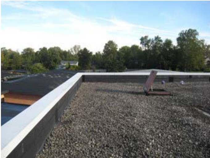
Ballasted Roof at 1988 Addition
