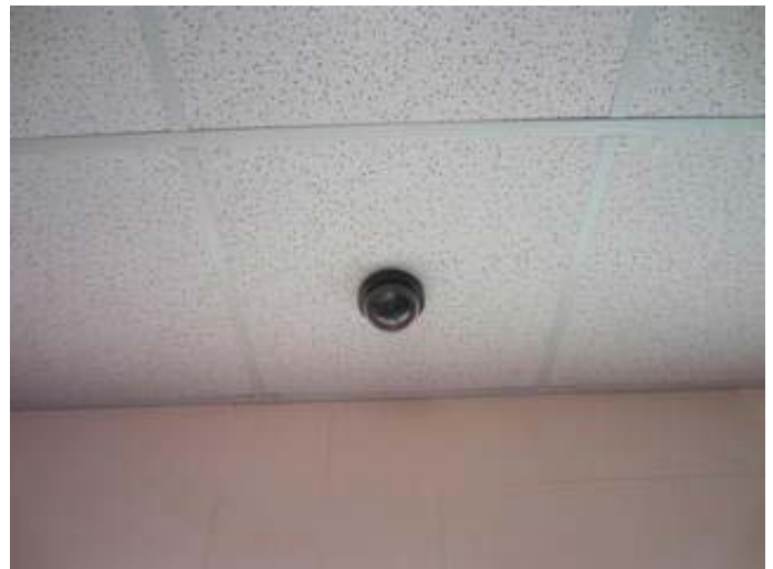
Security System CCTV Camera
