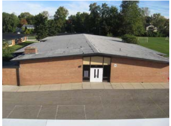
Membrane Roof at 1968 Addition
