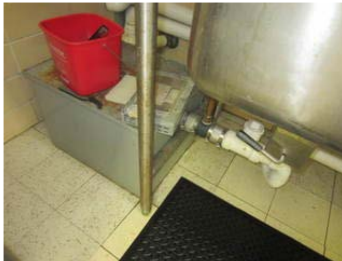
Kitchen Grease Trap Interceptor
