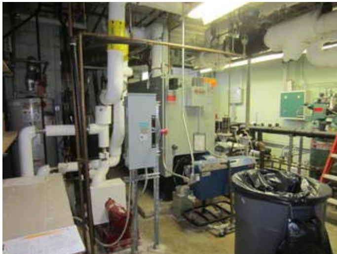
Natural Gas Fired Heated Water Boiler
