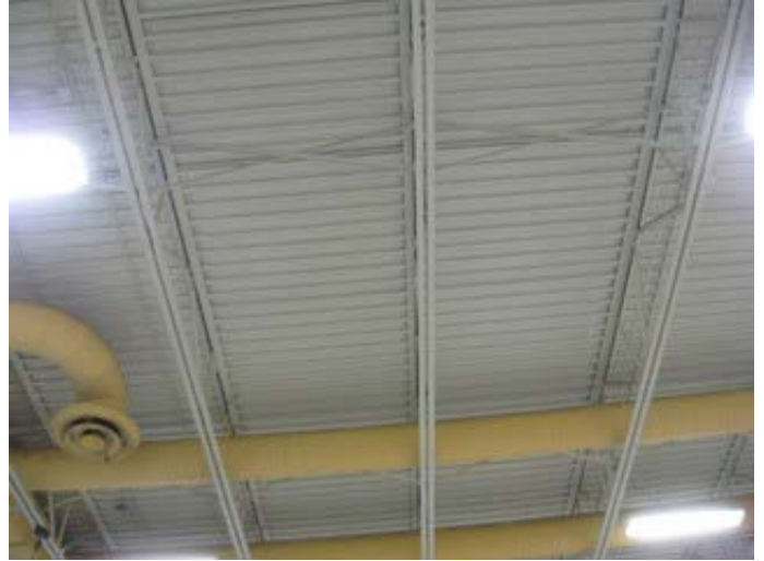
Steel Joist Structure
