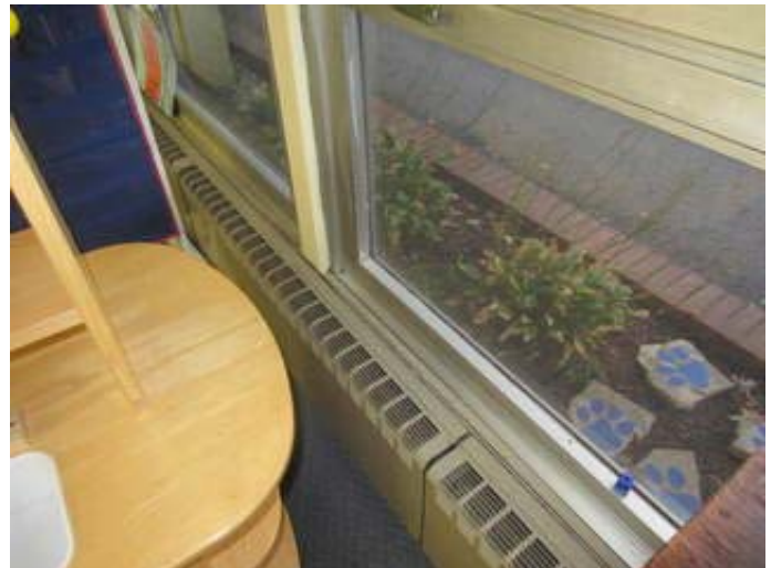
Heating Water Fin Tube
