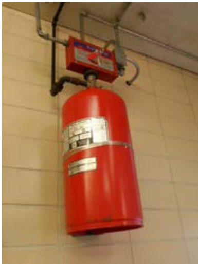
Compliant Wet Chemical Fire Suppression System
