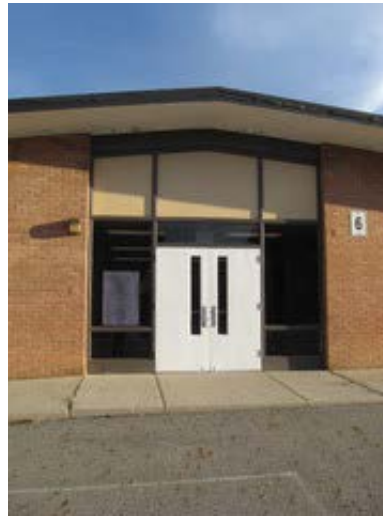
Hollow Metal Door with Transom and Sidelight
