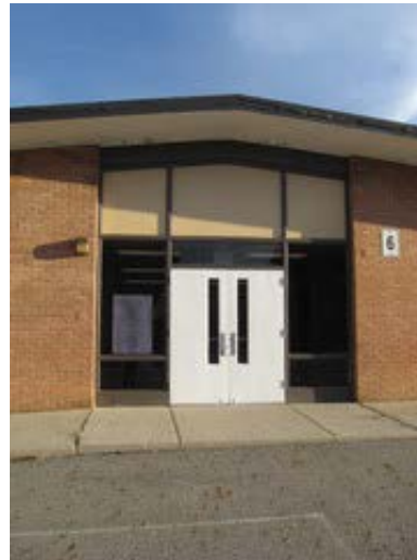
Hollow Metal Door with Transom and Sidelight
