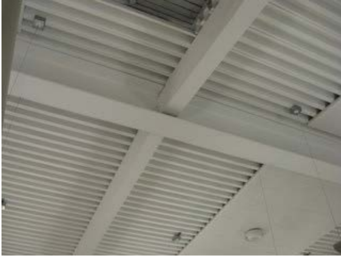
Structural Composite Metal Deck
